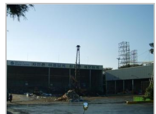
• Waste Treatment and Storage Facility
