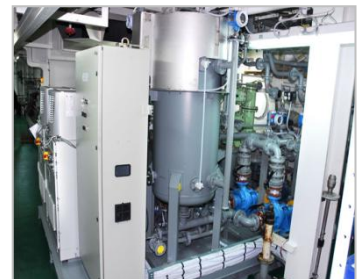
• Hi Ballast System
