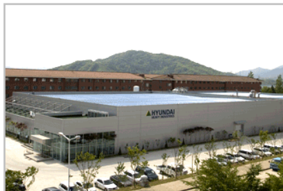
· Eumseong Solar cell-producing Plant
