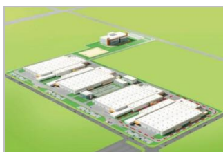
· Birds eye view of Hyundai Avancis CIGS solar module plant
