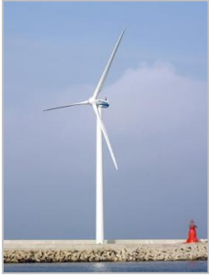
• 1.65MW wind turbine in the Ulsan shipyard
